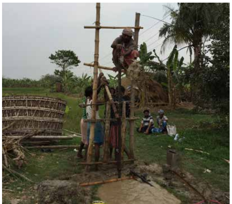
Drilling hand-pump technique, West Bengal, India (Photo: J. Adhikari)
