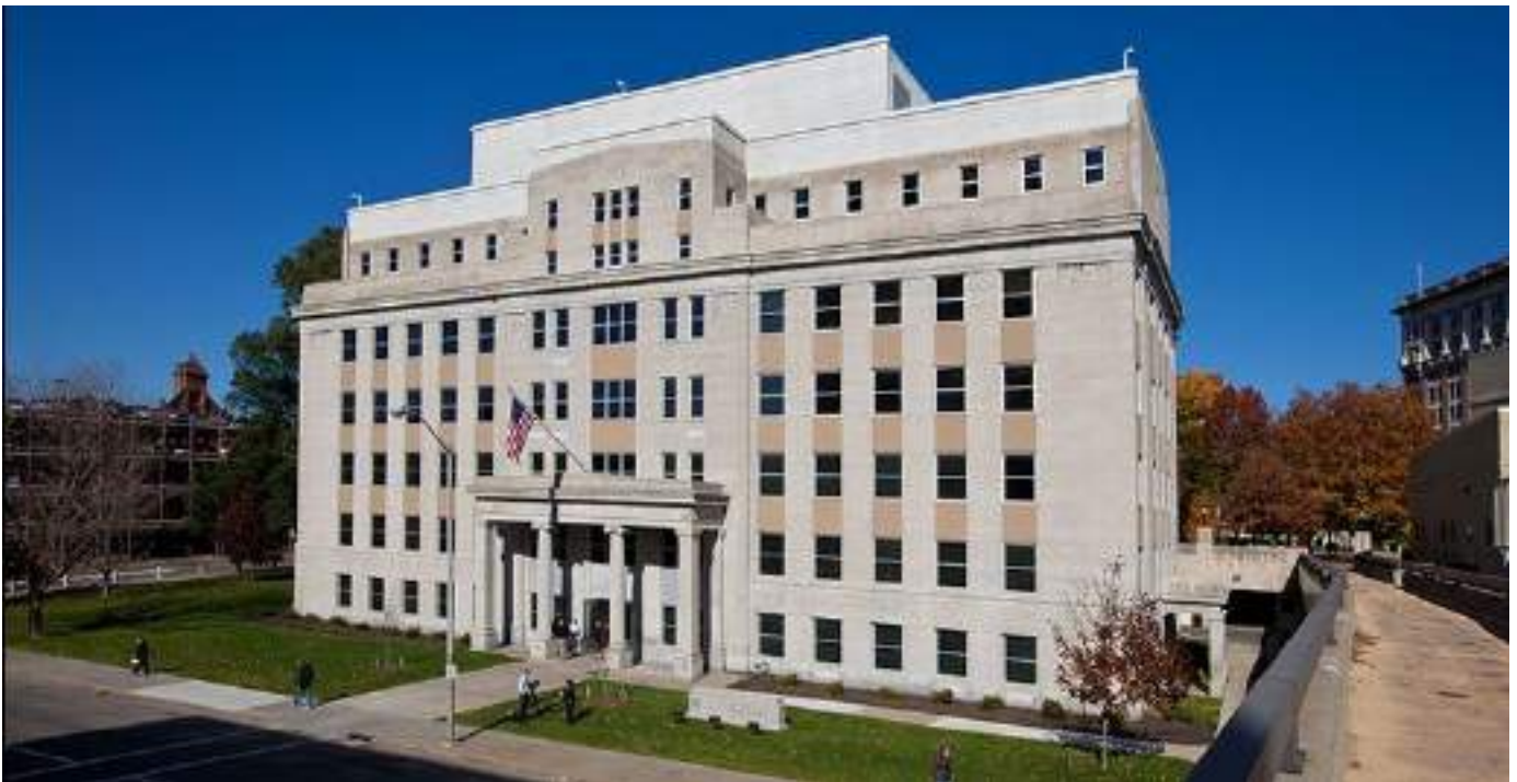
Broome County Family and County Courts, Downtown Binghamton
