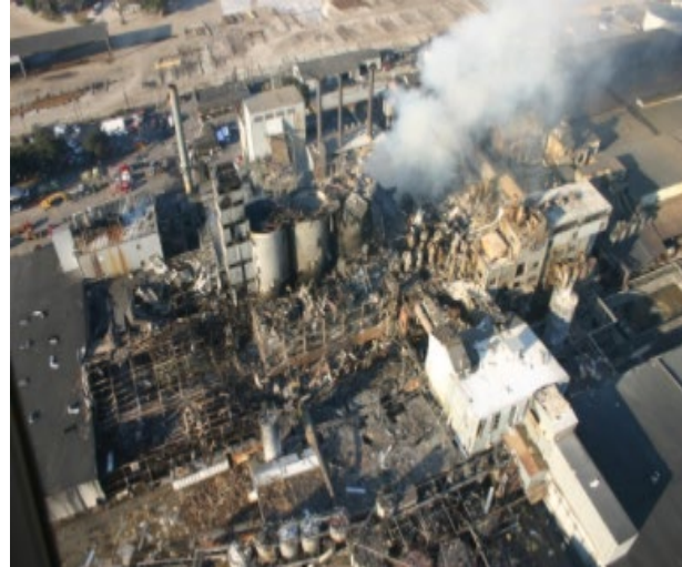
Figure 2: The 2008 Imperial Sugar explosion caused by excess sugar buildup. 14 people died, many more injured
